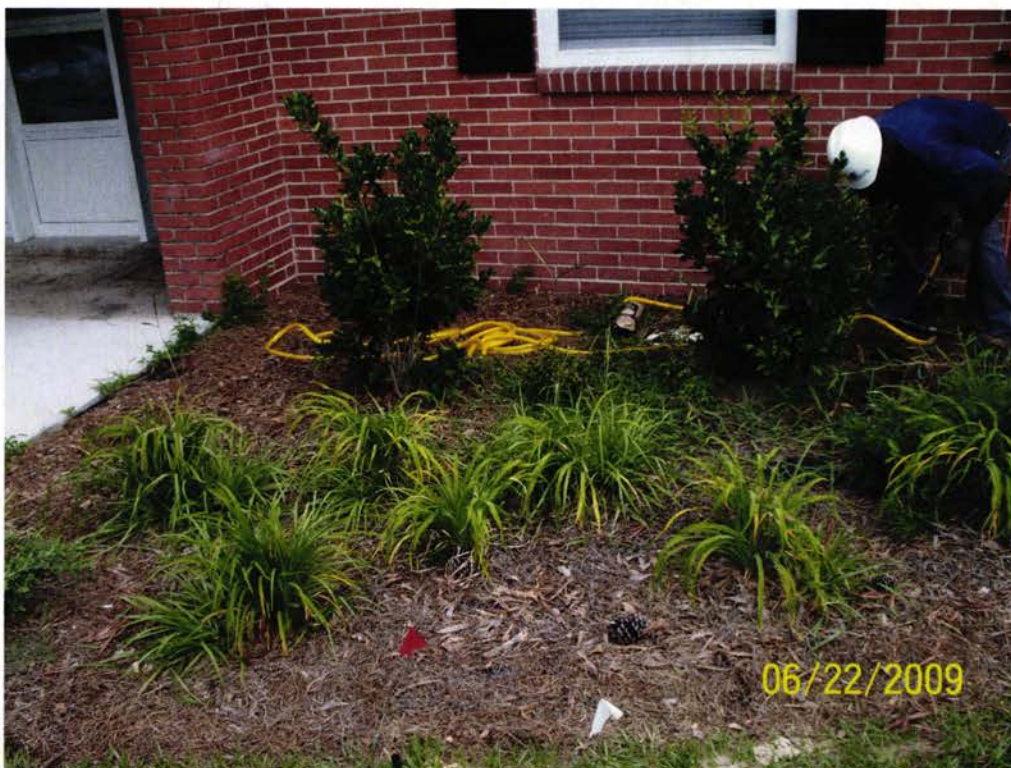
Picture 1: Location of UST 1138Iris prior to excavation.
